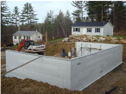
Completed foundation at the building trades site
